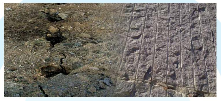
Besides the consistently applied production blasting performed in the mining and construction industries, controlled blasts and special custom blasts are needed for a variety of reasons including vibration and slope control. As BALEX Power Team we are proud to successfully complete and continue to provide services for special applications such as pre-split and smooth blasting in the mining, road construction, and dam and tunnel construction industries.
